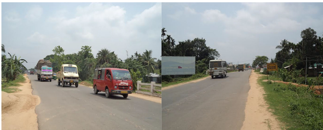
Fig. 1 A view of the study section on Assam–Agartala road (photos by the authors)
