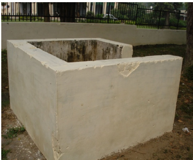
Fig. 3 Depot with masonry wall
