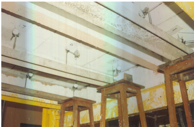
Fig. 4 Set-up of dial gauges under slab panels ( underside view )
