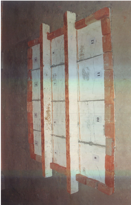
Fig. 6 Crack pattern in ferrocement panels with 0 % fly ash (underside view)
