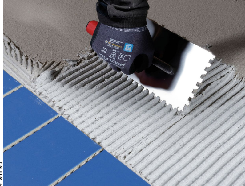
Application of the product MB FL 2K as a tile adhesive
