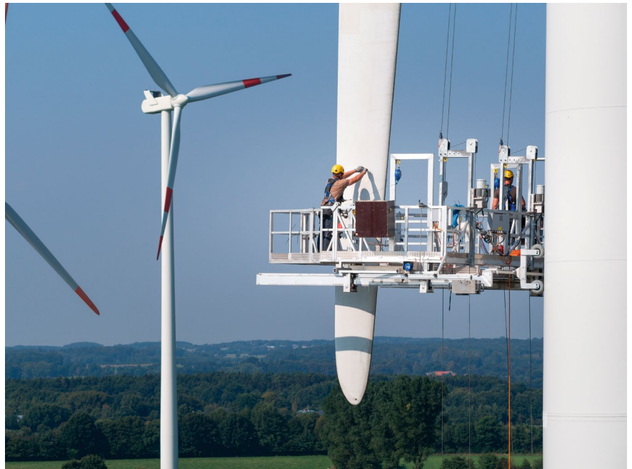
A new coating enables rotor blade leading edges to be repaired in a single step without a primer or filler.
