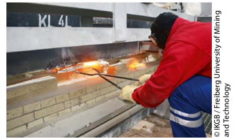
Industrial experiment on a glass melting furnace
