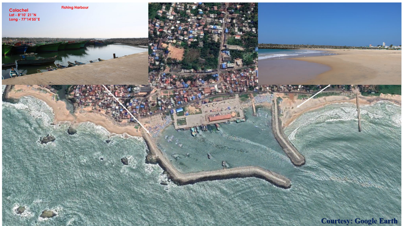
Fig. 10 Shoreline modification due to the construction of jetties and the accretional zone
