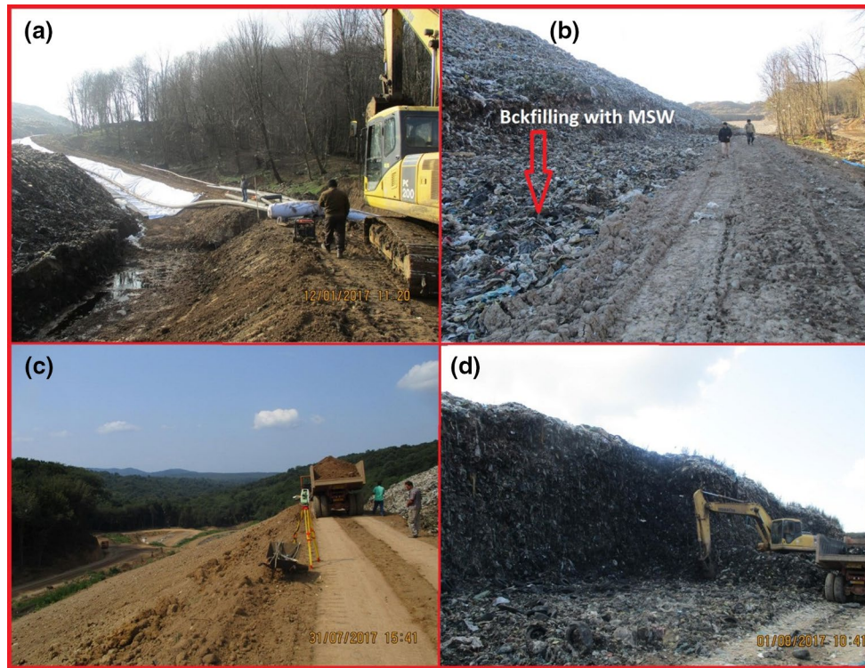
Fig. 20 Construction stage of side embankment covers
