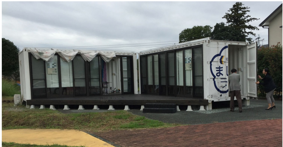
Fig. 6 Shipping containers serving as a community center in Mashiki town, near Kumamoto. Photograph by the author, October 2017
