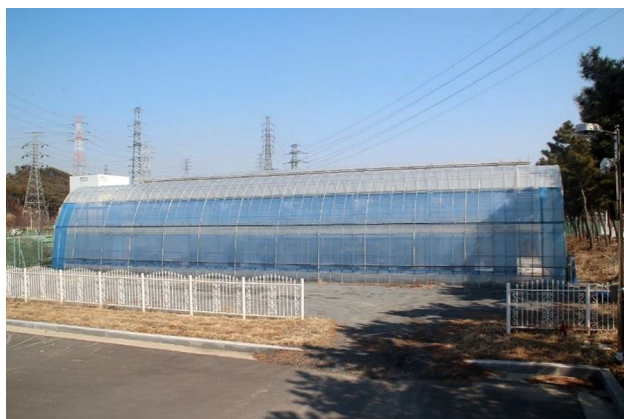
Fig. 1 A double-span arch-type plastic house (34.4 W × 30.0 L × 5.7 H, m) used for Irwin mango cultivation located at Boryeong, Korea
