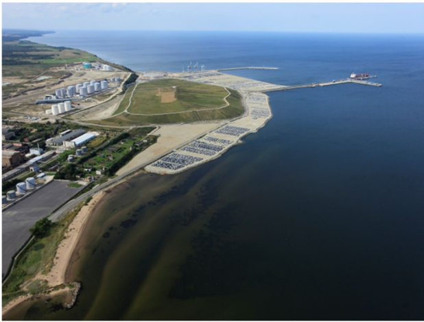
Fig. 18 Sillamäe Tailing Pond and Sillamäe Port, Spring 2012, Three years after completion of remediation. An Industrial Zone and transportation hub for road, sea, and railway. Remediation Detail Design and construction cost approximately EUR 21 million
