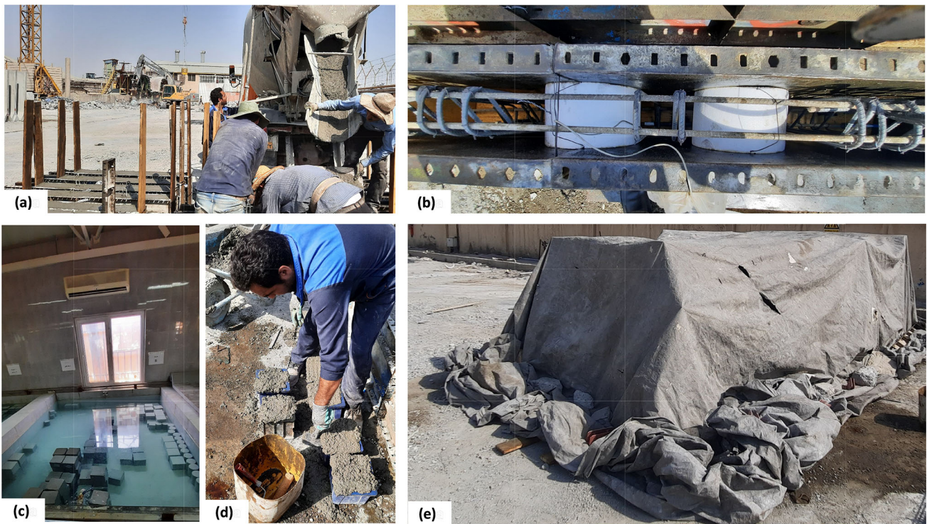
Fig. 2 Construction of specimens: a concrete casting; b polystyrene cylinders; c curing tank with cubic concrete samples; d cubic concrete samples; e curing beams under steam
