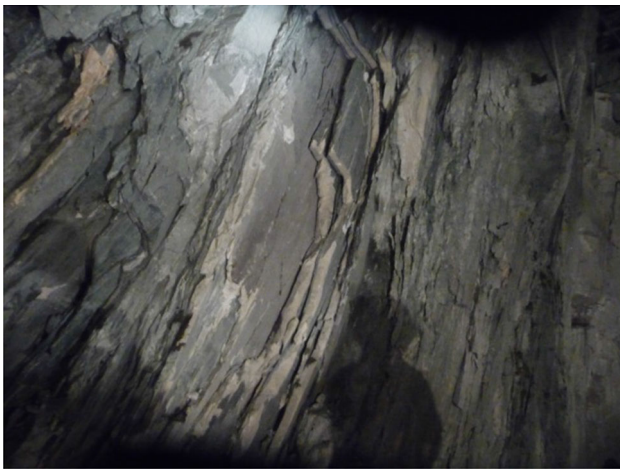
Fig. 4 The geological condition exposed
