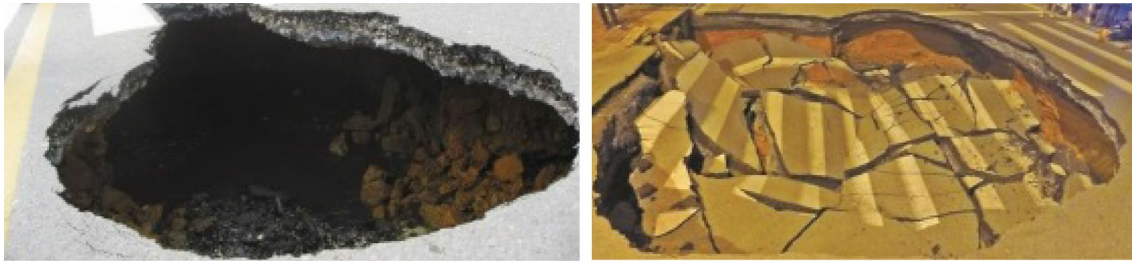
Fig. 11 Ground subsidence shape caused by shield tunnel face instability
