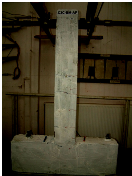
Fig. 2 General view of experimental stand element C3C–BM–AF after retrofit with crack pattern [16]
