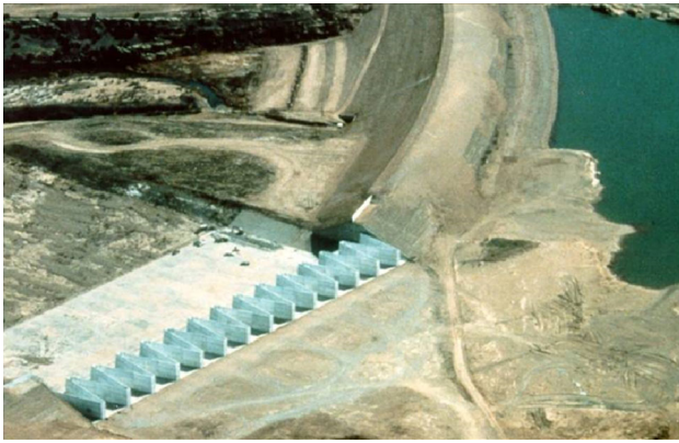
Fig. 3 Constructed labyrinth weir of Ute Dam
