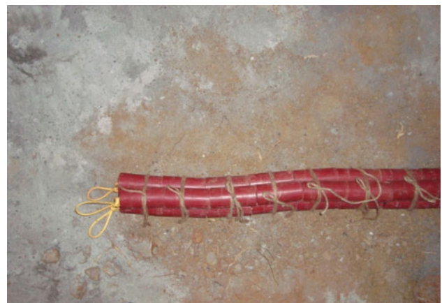
Fig. 9 Preparation of explosive before charging
