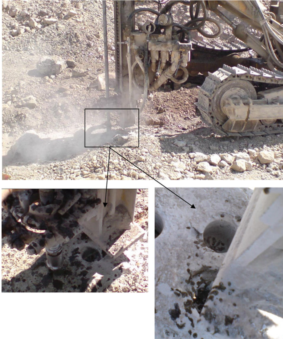
Fig. 2 Drilling the 10 cm sample holes
