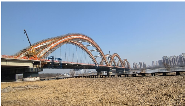
Fig. 5 General view of the bridge
