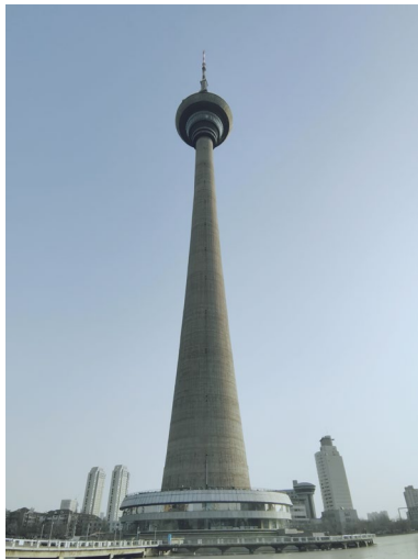
Fig. 9 The super-high-rise building
