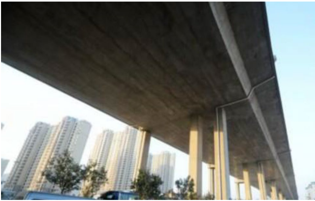
Fig. 13 Photograph of the actual bridges
