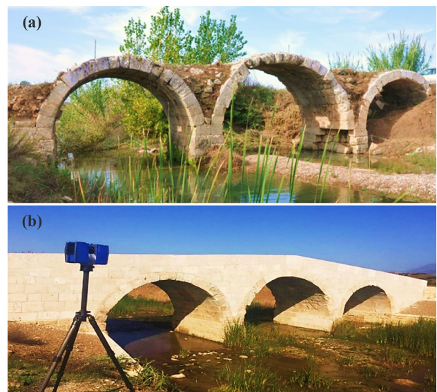
Fig. 1 Sillyon Bridge a before and b after restoration (downstream direction)
