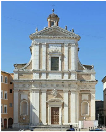
Fig. 2 View of San Giovanni from Corso della Repubblica before the 2016 Central Italy earthquake [18]
