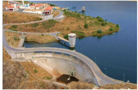
4 - Bouçã dam (crown length: 175m; height: 63m)
