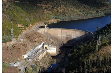
6 - Aguieira dam (crown length: 400m; height: 89m)
