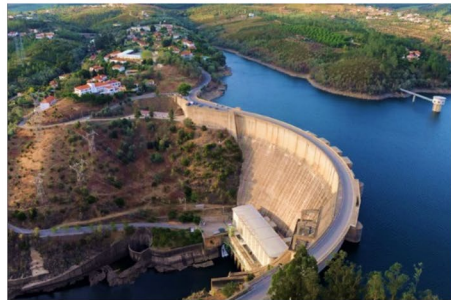
5 - Castelo do Bode dam (length: 402m; height: 115m)
