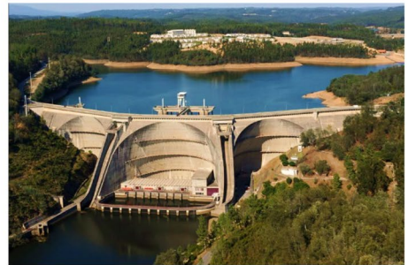
6 - Aguieira dam (crown length: 400m; height: 89m)
