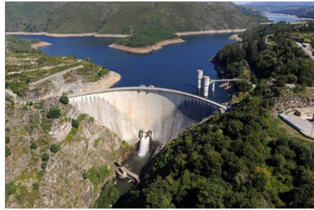
3 - Santa Luzia dam (crown length: 178m; height: 76m)
