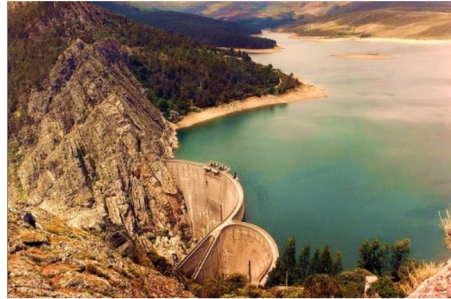
5 - Castelo do Bode dam (length: 402m; height: 115m)
