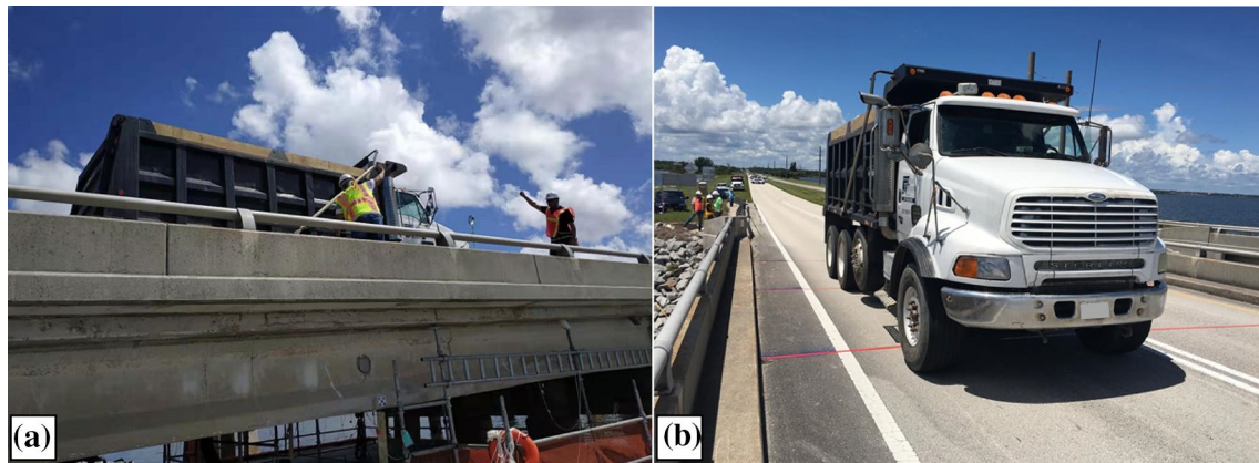
Fig. 10 Truck loading on the bridge
