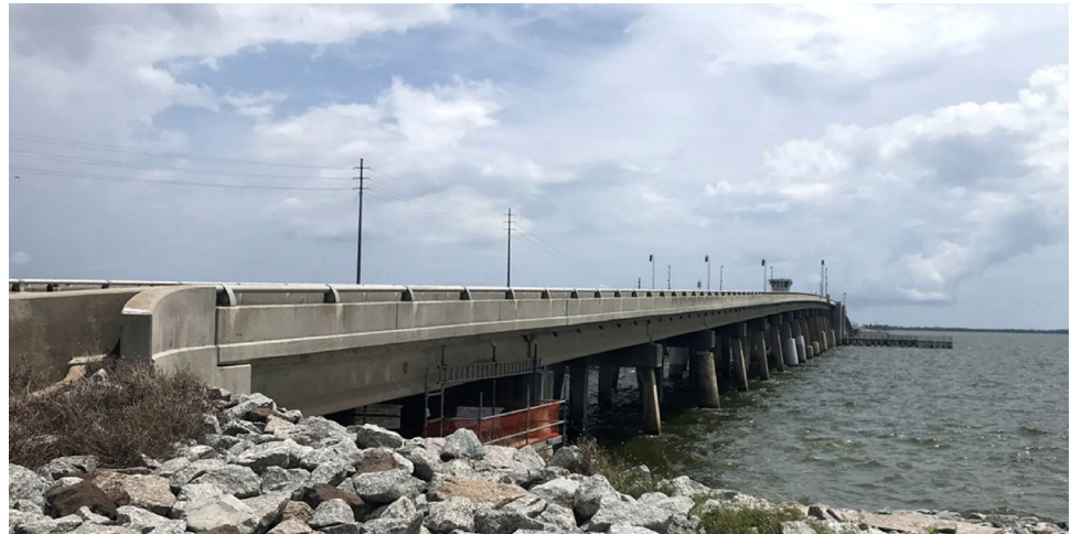
Fig. 6 The pre-stressed concrete highway bridge in this study
