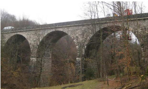
Fig. 10 View of the Gresal Bridge [7]
