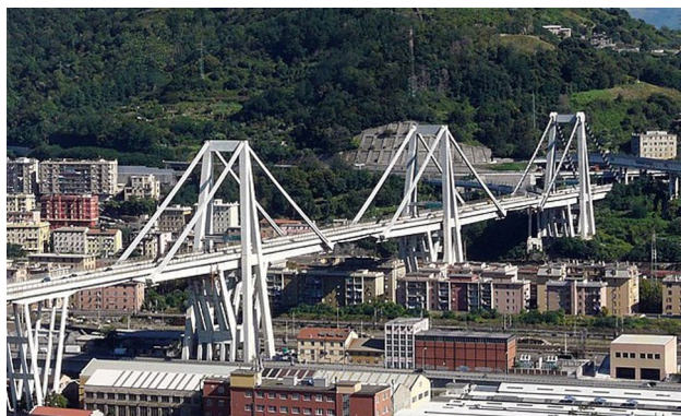
Fig. 1 The Polcevera Viaduct before the collapse of the first balanced system on the left (namely pier 9)
