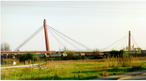
Fig. 12 The Indiano Cable-Stayed Bridge, Florence, Italy [9]
