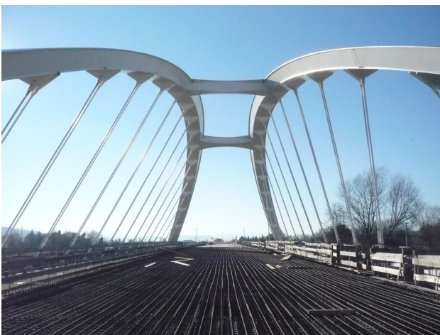
Fig. 14 The bridge on the Potenza river [11]
