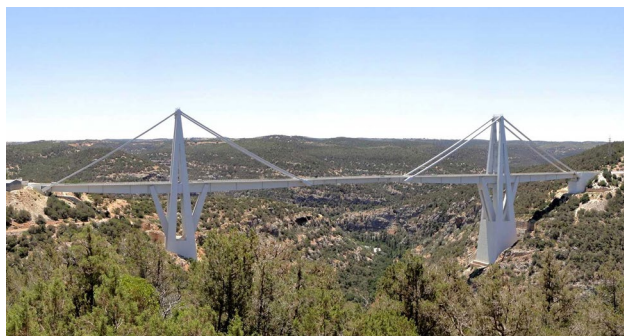
Fig. 3 The bridge over the Wadi al-Kuf in Libya
