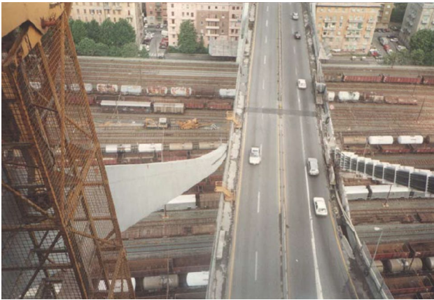
Fig. 5 Polcevera Viaduct: new strands on pier 11 [2]
