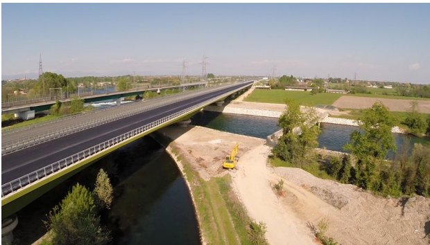
Fig. 13 View of the Adda Viaduct [10]
