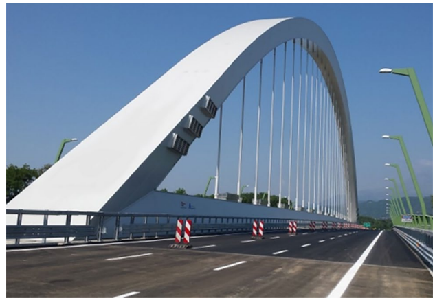
Fig. 16 General view of the suspended arch steel bridge [13]
