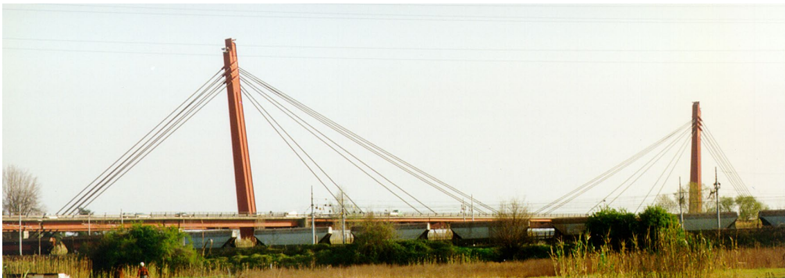
Fig. 1 The Indiano Cable-Stayed Bridge, Florence, Italy
