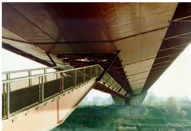
Fig. 6 The walkway for pedestrians and bicyclists suspended to the girder
