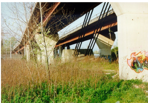
Fig. 4 One of the anchor stays, composed of two sets of three cables, with its external anchorage
