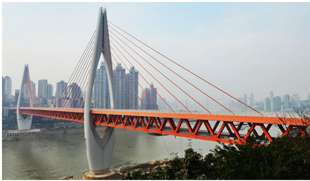
Fig. 1 Chongqing Dongshuimen Yangtze River Bridge, China, ( http://www.crbbg.com )
