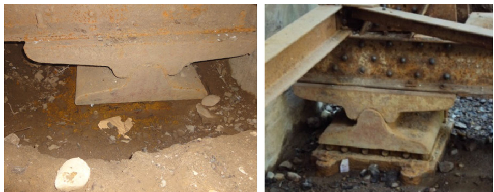
Fig. 7 Bearings before retrofitting and after retrofitting
