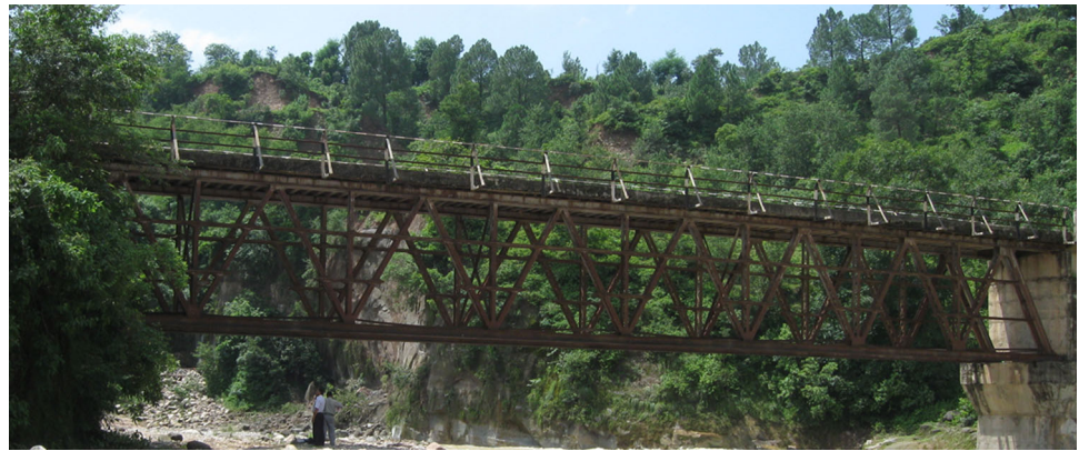
Fig. 1 Steel truss bridge of span 47.90 m over Bathu Khad
