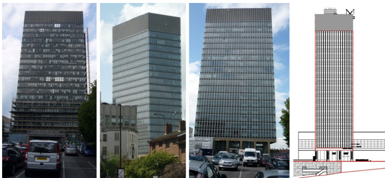
Fig. 1 Views of Arts Tower: during retrofit ( left ), after retrofit ( middle pair ) and east elevation
