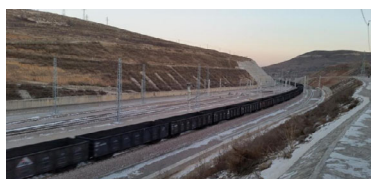
Fig. 1 Shuohuang Railway in K3.
