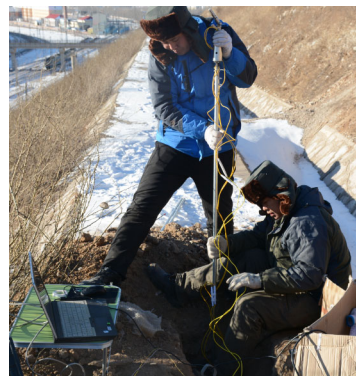
Fig. 12 Installation photo of the FBG sensors.
