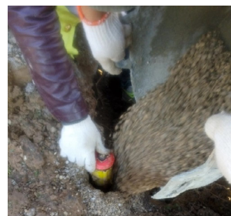
Fig. 11 Backfilling of the borehole.
