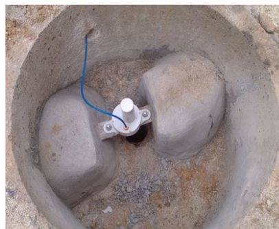
Fig. 7 Field installation of displacement sensor.
