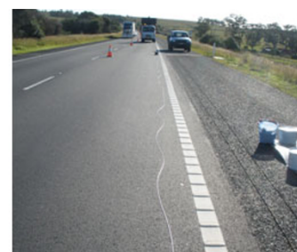
Unspooling the temp cable
