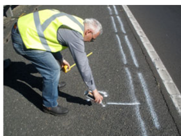
Marking out the site
