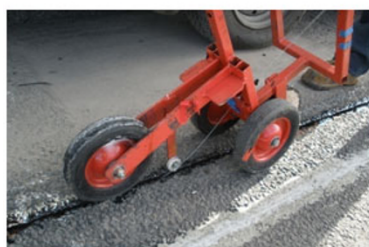
Feeding the strain cable into the slots
