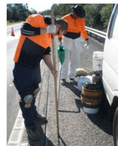
Using a gauge stick to ensure the cable is embedded at the correct depth
