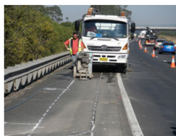
Saw cutting the slots
