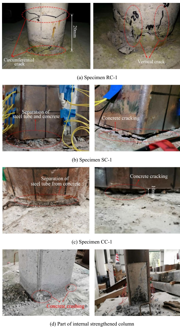
Fig. 5 Failure modes of the specimens
