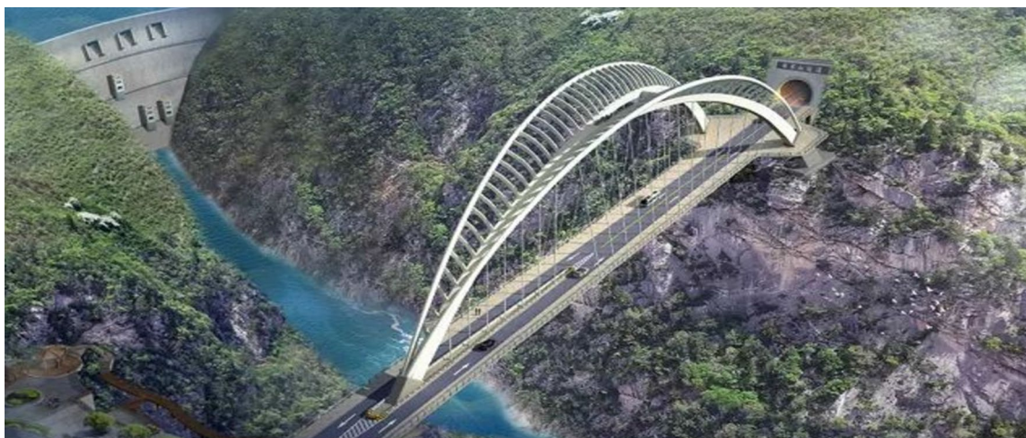
Fig. 1 3Dmodel diagram of the spatial Y-shaped tied arch bridge
