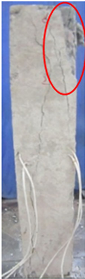
Fig. 4 Typical failure of RC columns without strengthening
