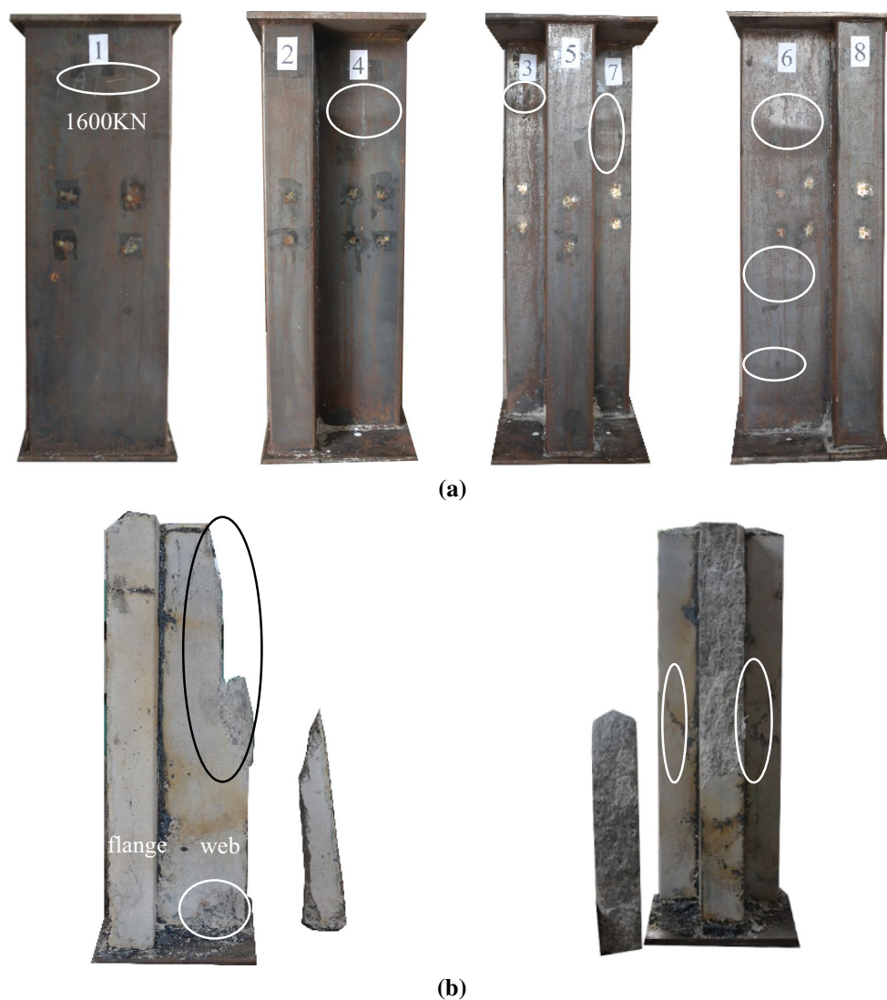
Fig. 4 Failure mode of specimen TA1. a Local buckling of steel tube and b concrete damage
