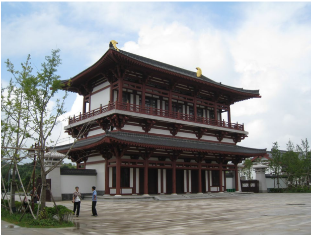
Fig. 1 Typical steel traditional-style buildings
