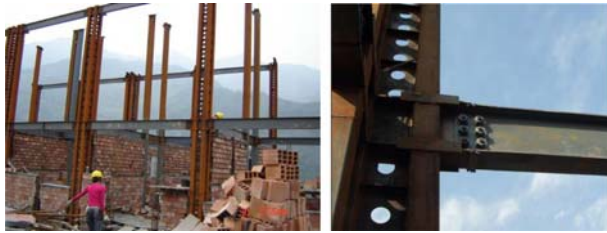
Figure 2. Photo of an SCFST column structure.
