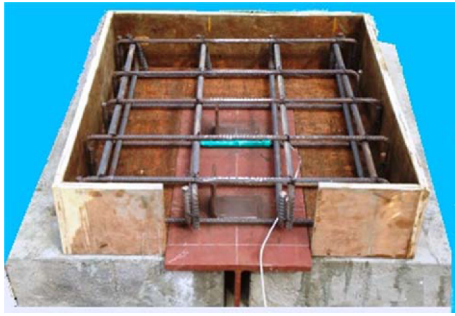
Figure 5. Construction of concrete formwork.
