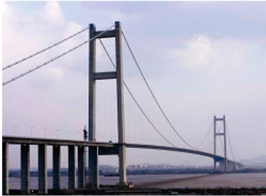
Figure 1. View of the Runyang Suspension Bridge.
