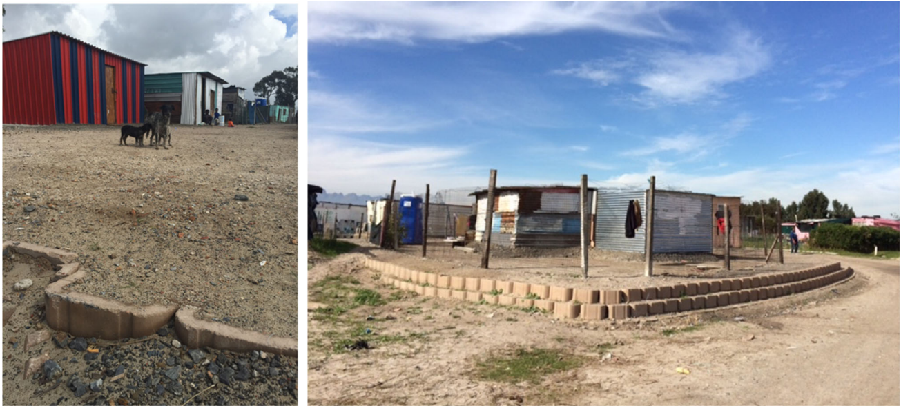
Fig. 2 Examples of the gravel platforms that have been constructed in Green Park informal settlement
