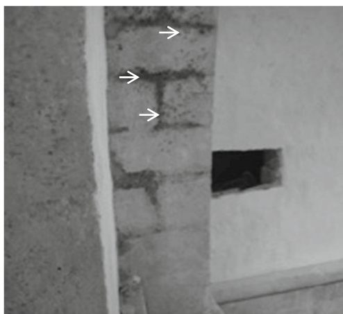
Fig. 3 Wall from Les Salles-Lavauguyon church France, colonized by fungi. The arrows indicate areas of high colonization
