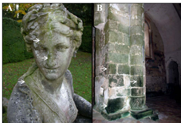
Fig. 2 Stone surface of a sculpture from the park of Courances castle France (a), and of pillars from the “Les Salles-Lavauguyon” church France (b), colonized by algae. The arrows indicate areas of high colonization
