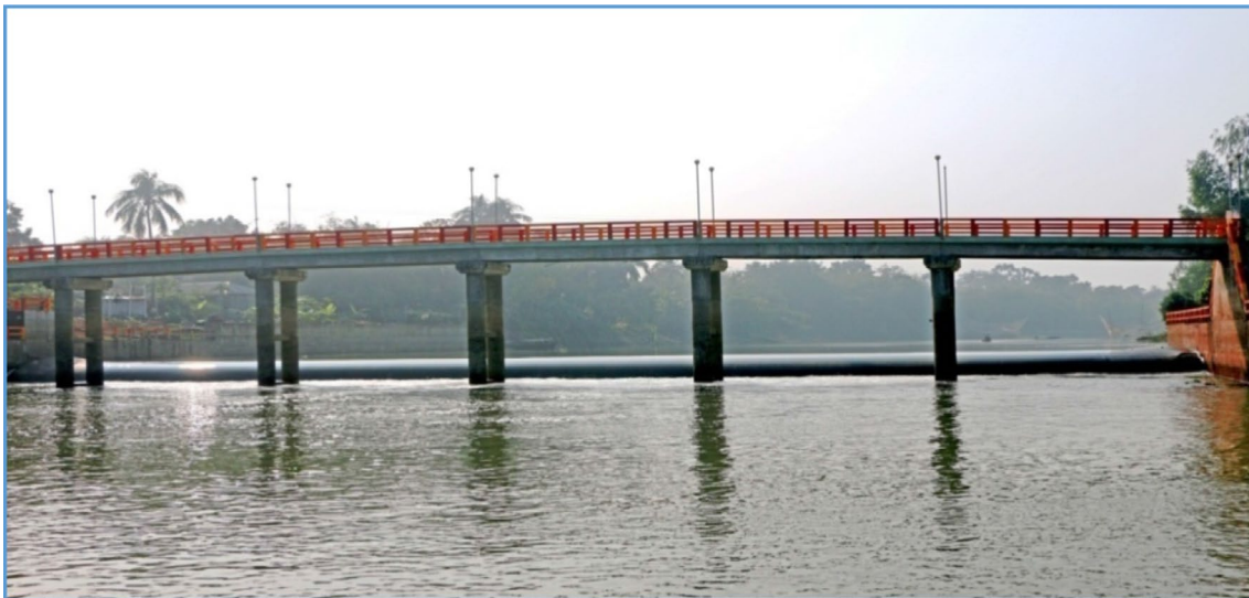
Fig. 3 A Rubber dam across the river Barnai at Jagodishpur, Puthia, Rajshahi
