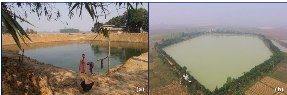
Fig. 4 Re-excavated ponds- a Konnyapara (Re-excavated area 1.09 acre), Niamatpur, b Kushumkunda (Re-excavated area 17 acre), Porsha
