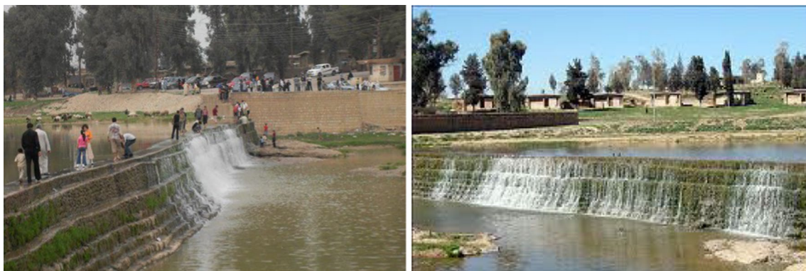
Fig. 2 Front and side view of the stepped weir
