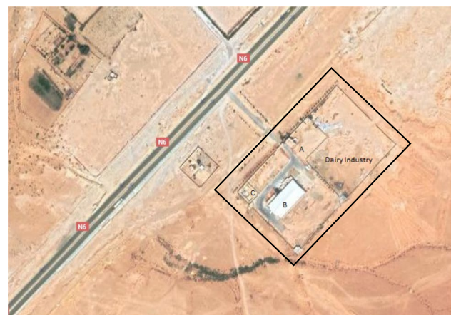
Fig. 1 Satellite view of location and structure of the studied dairy industry (Ouakda-Bechar, Southwest of Algeria) (Google maps 2020). A administration block; B manufacturing workshop; C basin for collection and disposal of the dairy effluents
