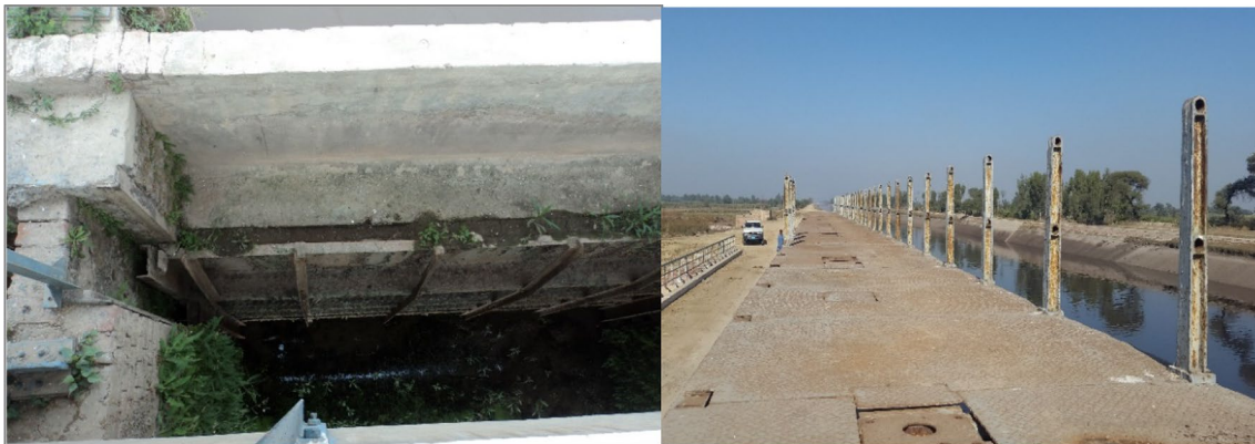
Fig. 9 One of the gates of BS Link escape (L); and hedge without operating motors (R)
