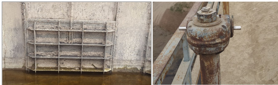
Fig. 11 SMB Link escape gate (left) and its operating mechanism
