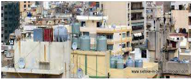
Fig. 4 Roof water tanks
