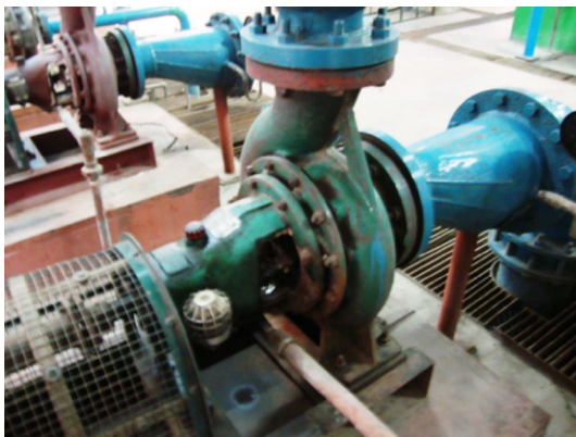
Fig. 5 Radial split case design pump—Design B
