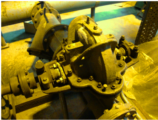
Fig. 4 Horizontal split case design pump—Design A
