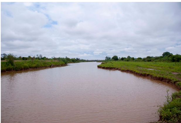
Fig. 6 Canalization of the Bañado La Estrella in the Sombrero Negro community with a containment barrier to the left. Photo taken by the first author
